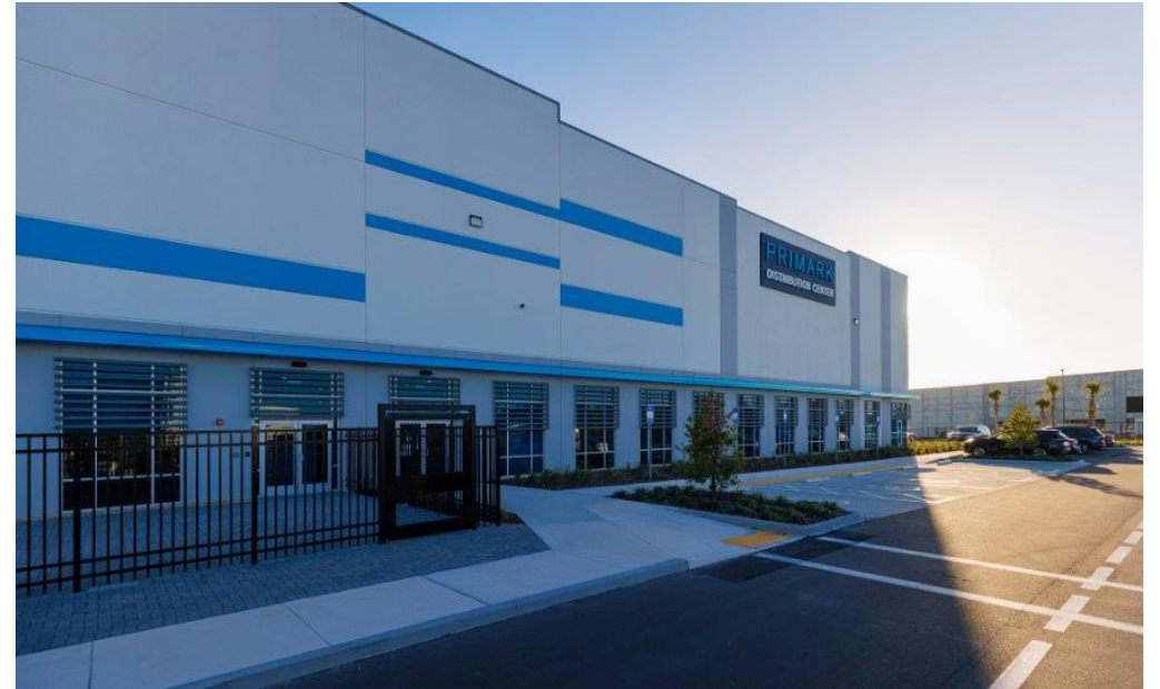
New distribution centre in Jacksonville, Florida
