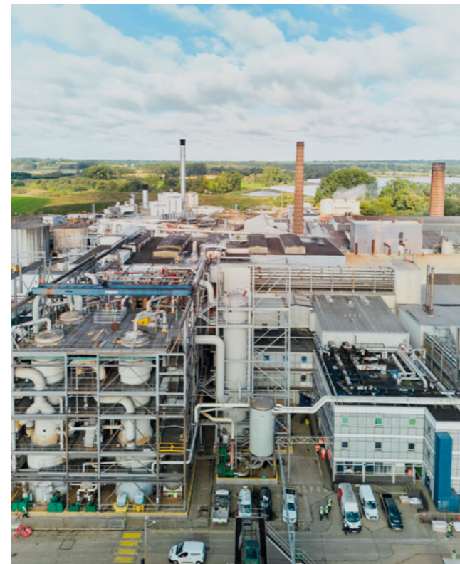
A new evaporator installed at British Sugar's factory in Wigginton as part of a project to reduce site emissions
